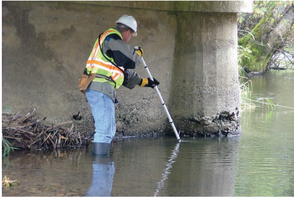
Figure 11.3.3 Wading Inspection
