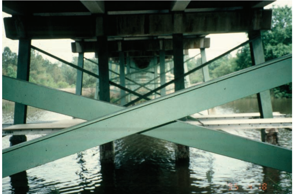
Figure 11.3.16 Steel Pile Bent
