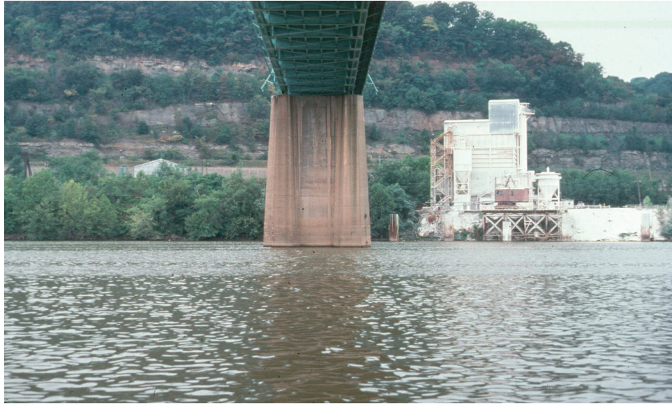
Figure 11.3.18 Column Pier with Solid Web Wall
