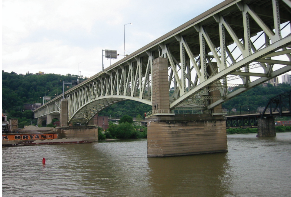
Figure 11.3.2 Liberty Bridge over Monongahela River
