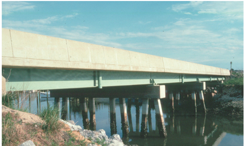
Figure 11.3.17 Concrete Pile Bent
