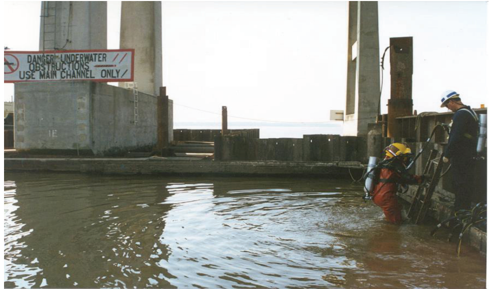
Figure 11.3.50 Diving Inside a Cofferdam
