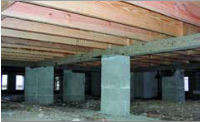
Treated Southern Pine 4x6 sill beams are supported by concrete block piers on a continuous spread footing.
