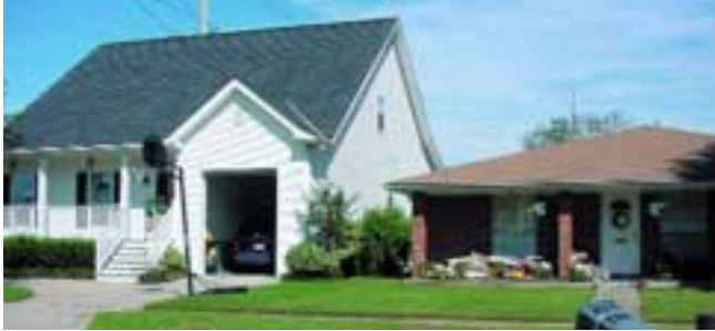
Tropical Storm Isidore flooded the slab-on-grade home on the right. The raised floor home on the left stayed dry.
