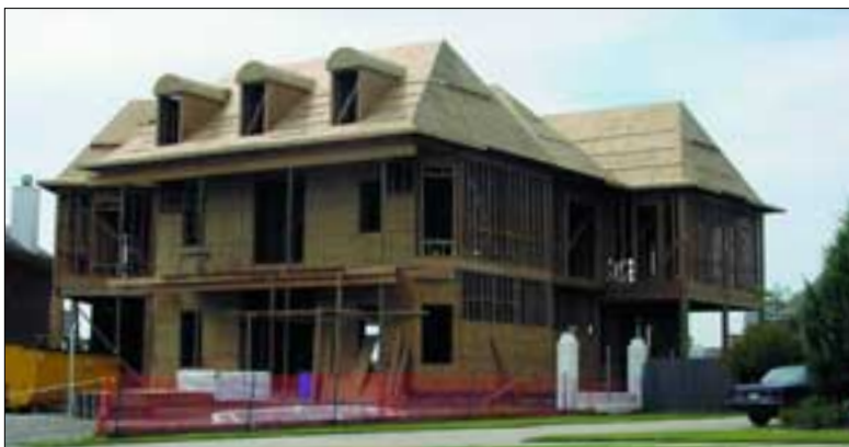
Optimum protection against Formosan termites is attained by using all pressure-treated Southern Pine kiln-dried after treatment (KDAT) lumber and sheathing for this 14,000 square-foot lakefront home in suburban New Orleans.
