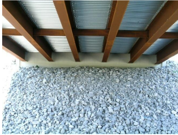
Figure 14 Photograph of a completed integral abutment.
