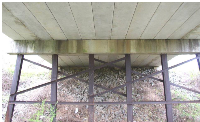
Figure 23 Pile bent with braced steel H-piles serving as both columns and foundations for the pier.
