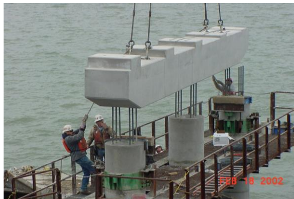
Figure 32 Example of a precast pier cap being used on a long viaduct bridge. The columns were cast-in-place with dowels projecting from the top of the columns. The dowels fit into pockets in the precast pier cap. The pier cap initially rested on collars around the tops of the columns. The collars were adjustable to facilitate leveling of the pier cap. Once the pier cap was set, grout was injected into the dowel pockets and the gap between the columns and the pier cap.
