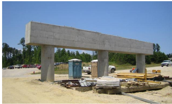
Figure 17 Typical multi-column pier with round columns and a prismatic pier cap.
