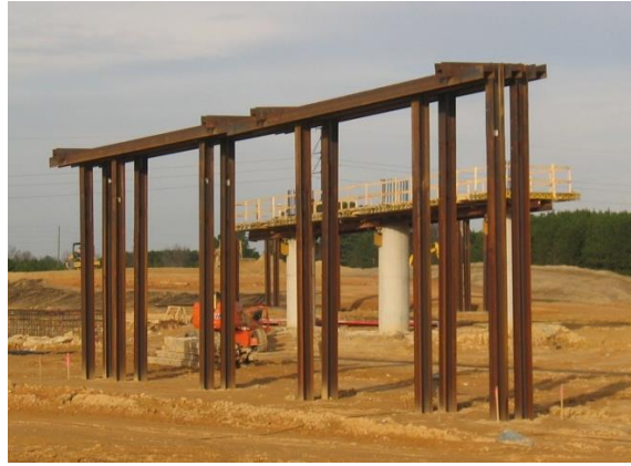
Figure 3 Driven steel H-piles arranged as the foundation for a conventional abutment. Later, MSE retaining walls will be built in front of these piles, and after that the abutment cap and backwall will be cast.
