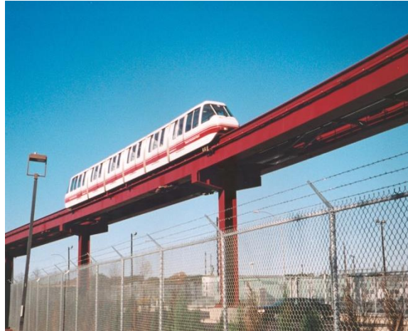
Figure 28 Steel single column hammerhead piers for a dual box girder automated people mover bridge.
