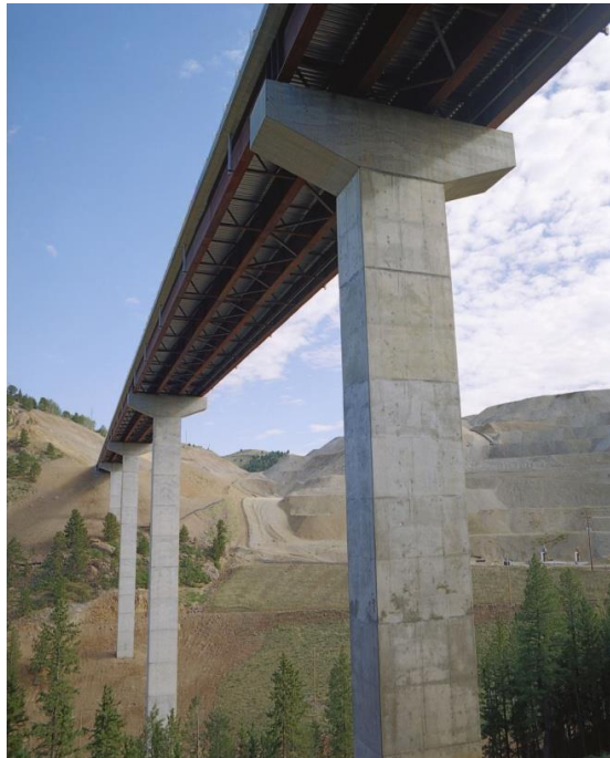
Figure 20 Single column hammerhead pier with very tall columns over a deep valley.
