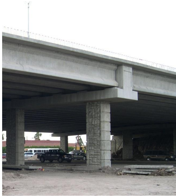
Figure 29 Inverted T pier cap in a multi-column pier.
