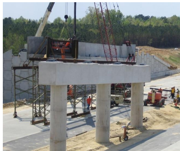
Figure 18 Typical multi-column pier with round columns and a stepped pier cap.
