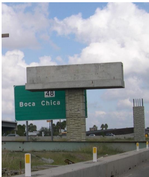
Figure 21 Single column hammerhead pier with an inverted T pier cap.
