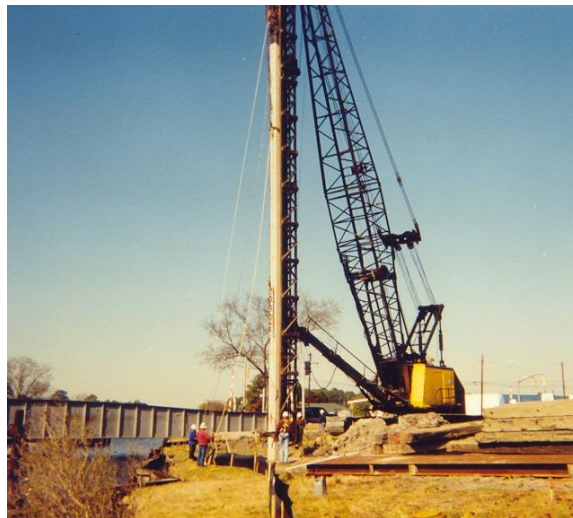
Figure 4 Driving of a precast concrete pile.
