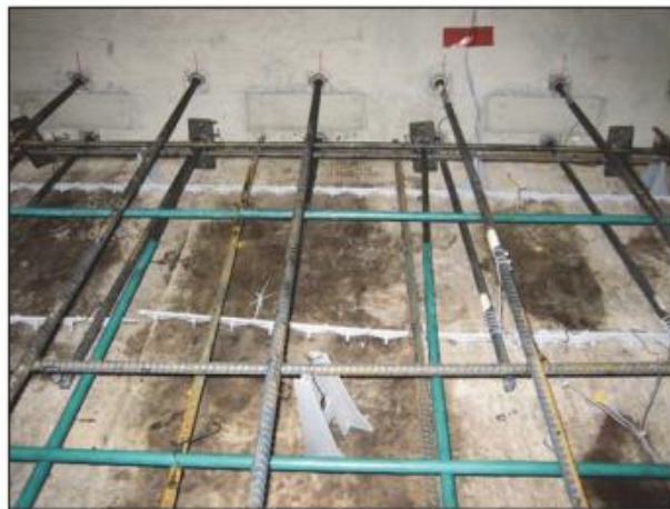
Figure 31. Form-face couplers for dowel anchorage.
