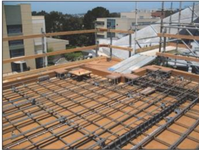
Figure 30. Confinement of a collector
