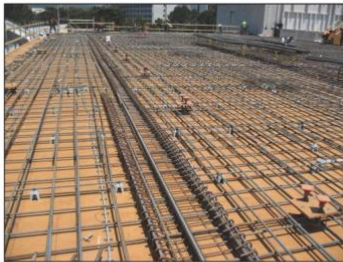
Figure 29. A long collector with confinement reinforcement
