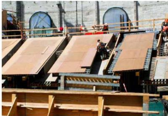
Figure 13. Historic Stadium Meets Modern Standards with Overlaid Plywood Forms
