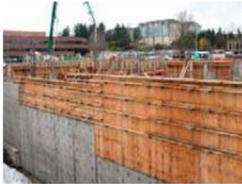
Figure 10. Engineered Wood Formwork is Cost-Effective, Customizable for Apartment Buildings
