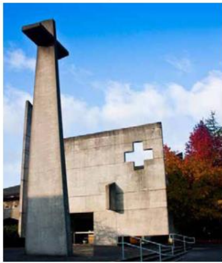
Figure 11. Subtle Architectural Expression Achieved with Simple, Practical Forming Approach
