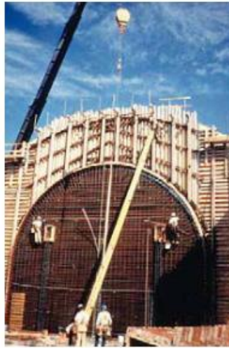
Figure 12. Engineered Wood Shapes State History: Wood Structural Panels Used to Form Massive Concrete Arches
