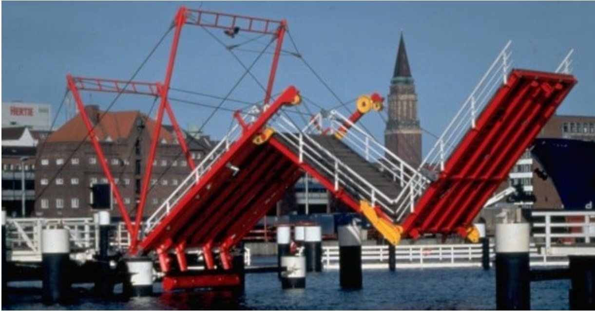
Figure 7. Folding Bridge
