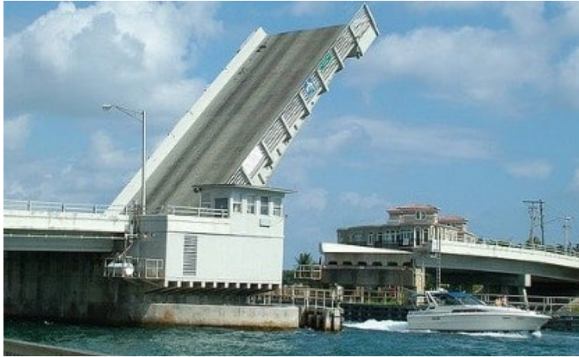
Figure 1. Single Leaf Bascule Bridge
