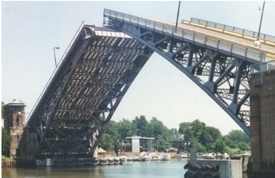
Figure 2. Double Leaf Bascule Bridge
