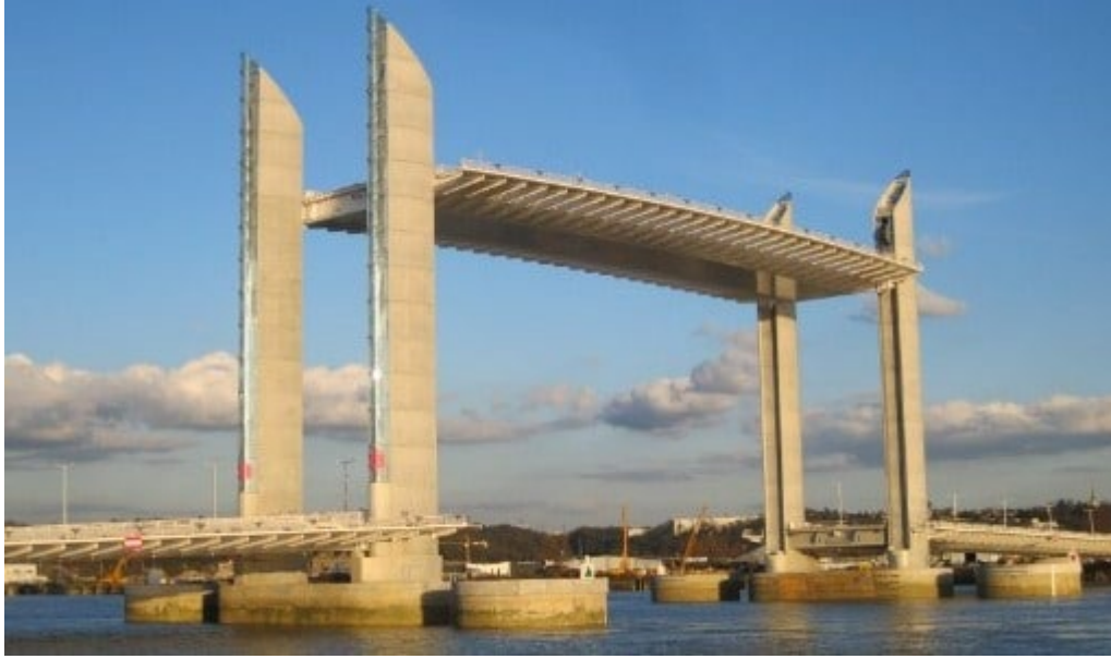
Figure 5. Vertical Lifting Bridge
