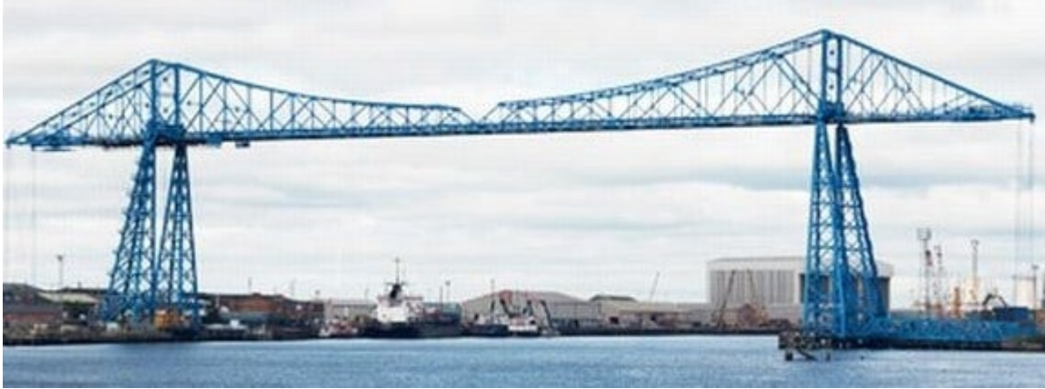
Figure 8. Transporter Bridge
