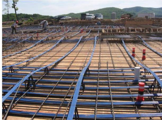
Figure 1. Post tension cables
