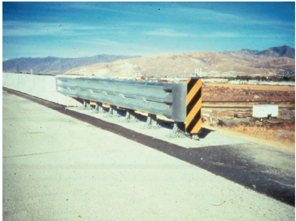
Figure 5.5.1 Bridge Safety Feature
