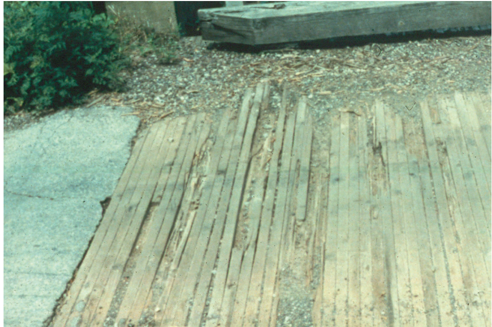
Figure 5.1.8 Wear and Weathering on a Timber Deck
