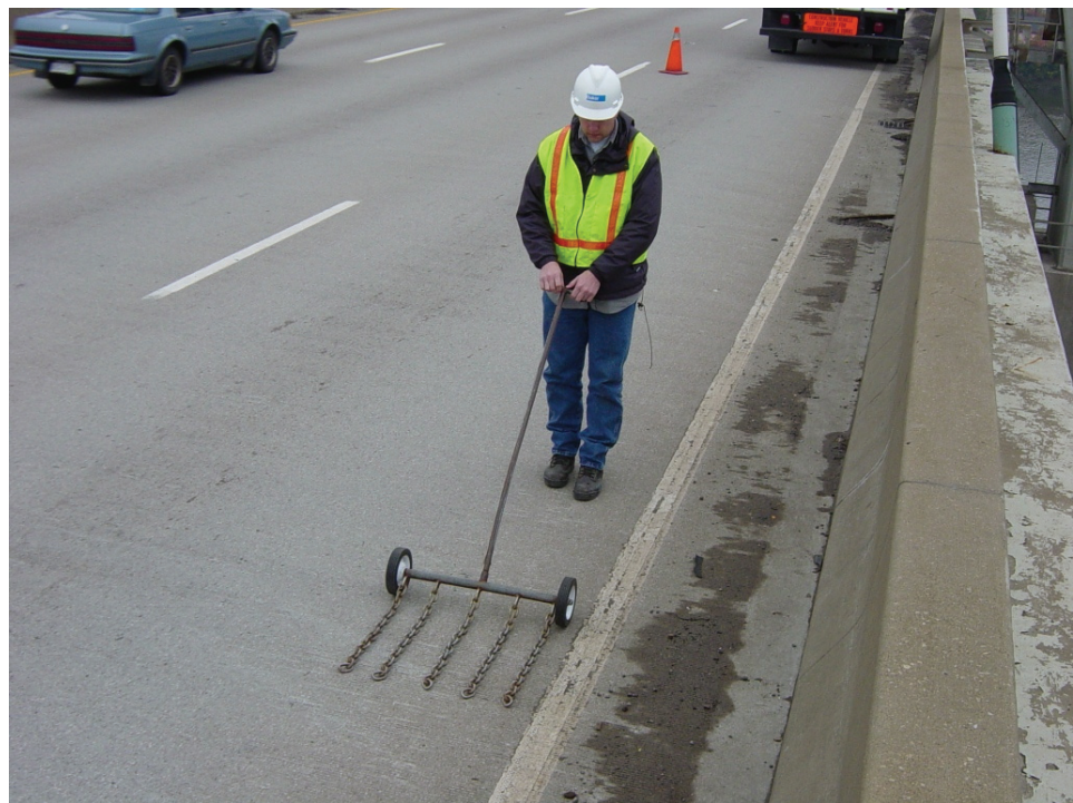
Figure 5.2.10 Sounding for Delaminated Areas of Concrete
