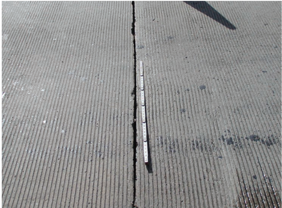
Figure 5.4.1 Formed Joint
