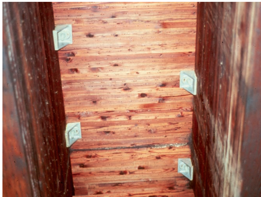
Figure 5.1.3 Glued-laminated Deck Panels
