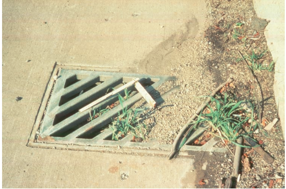
Figure 5.4.13 Bridge Deck Drain
