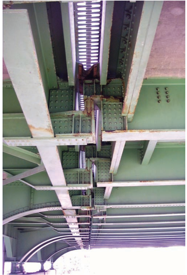
Figure 5.4.20 Support System under a Finger Plate Joint
