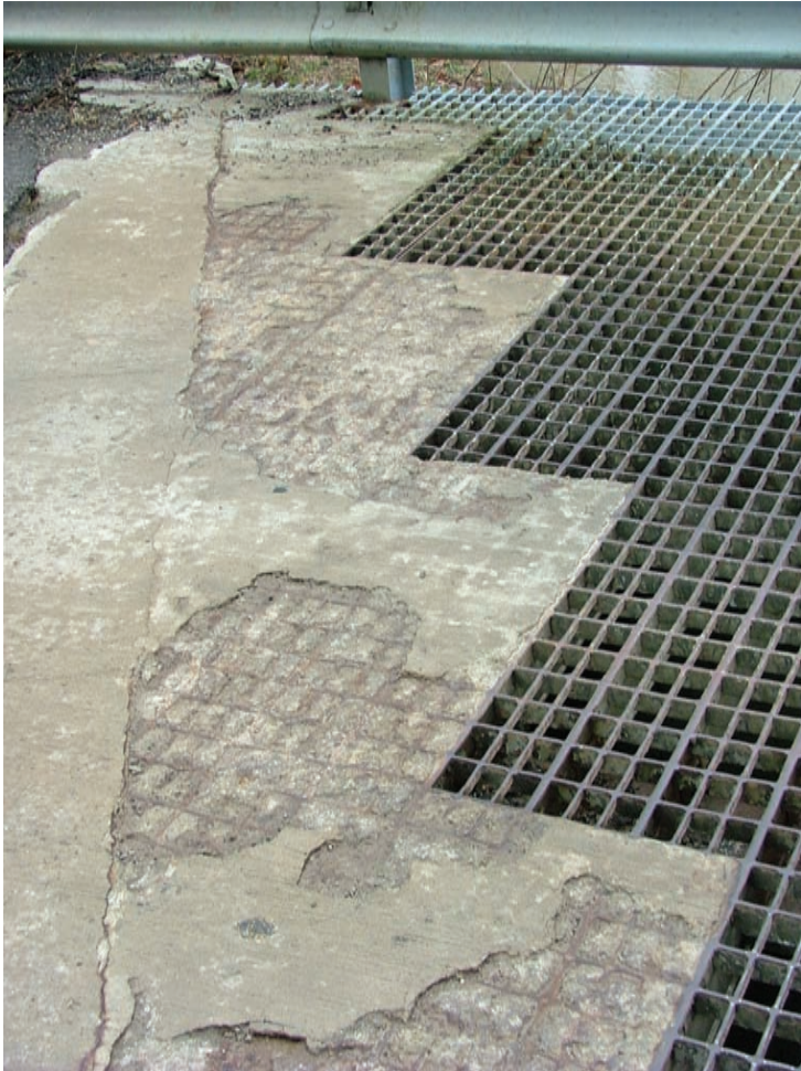
Figure 5.3.5 Filled and Un-filled Steel Grid Deck
