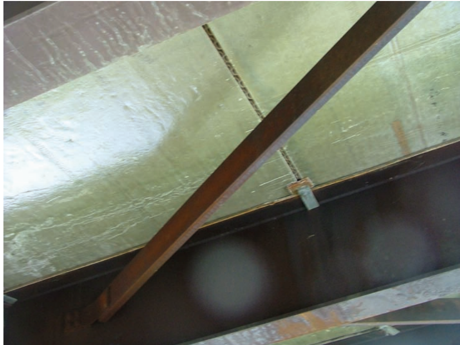
Figure 5.2.3 Fiber Reinforced Polymer (FRP) Deck
