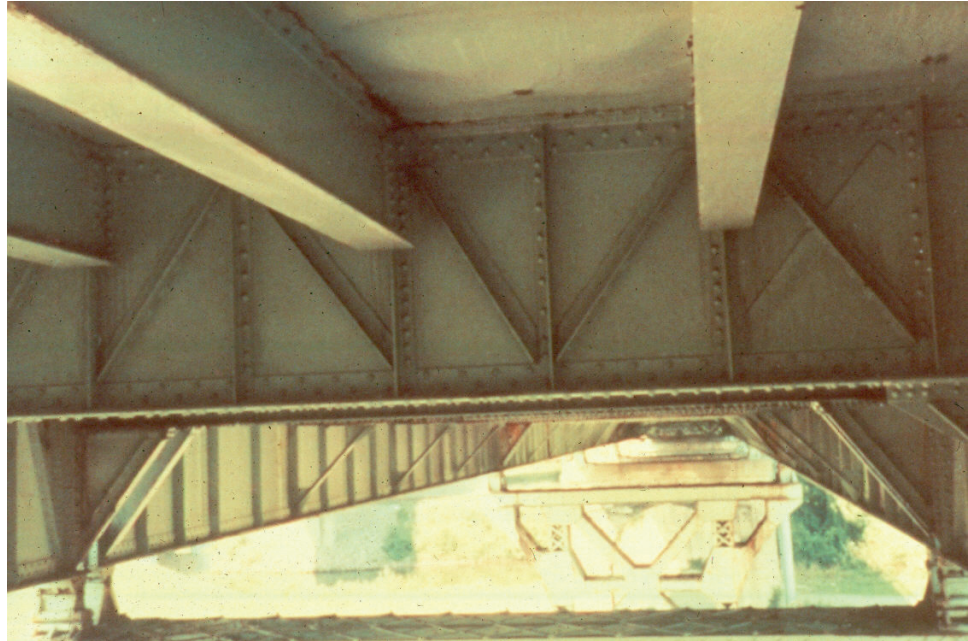
Figure 5.3.2 Underside View of Buckle Plate Deck
