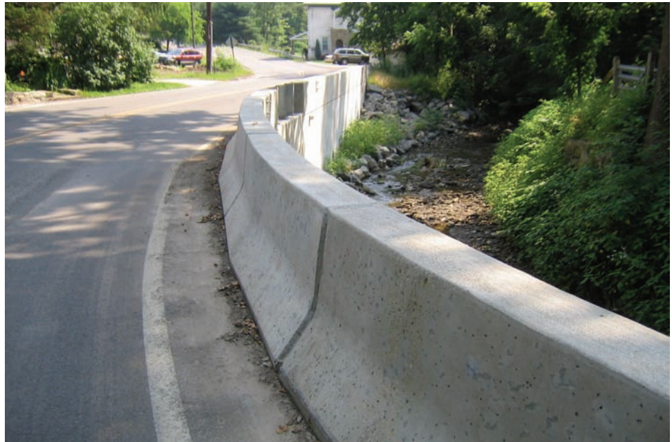
Figure 5.5.4 Acceptable Bridge Rail
