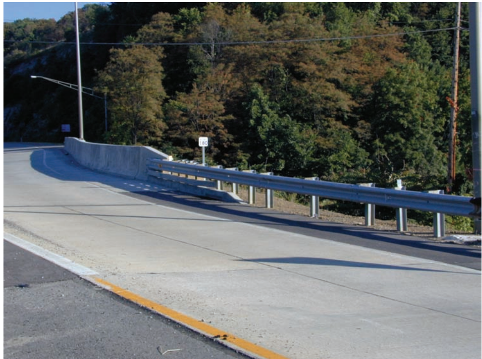
Figure 5.5.7 Approach Guardrail System
