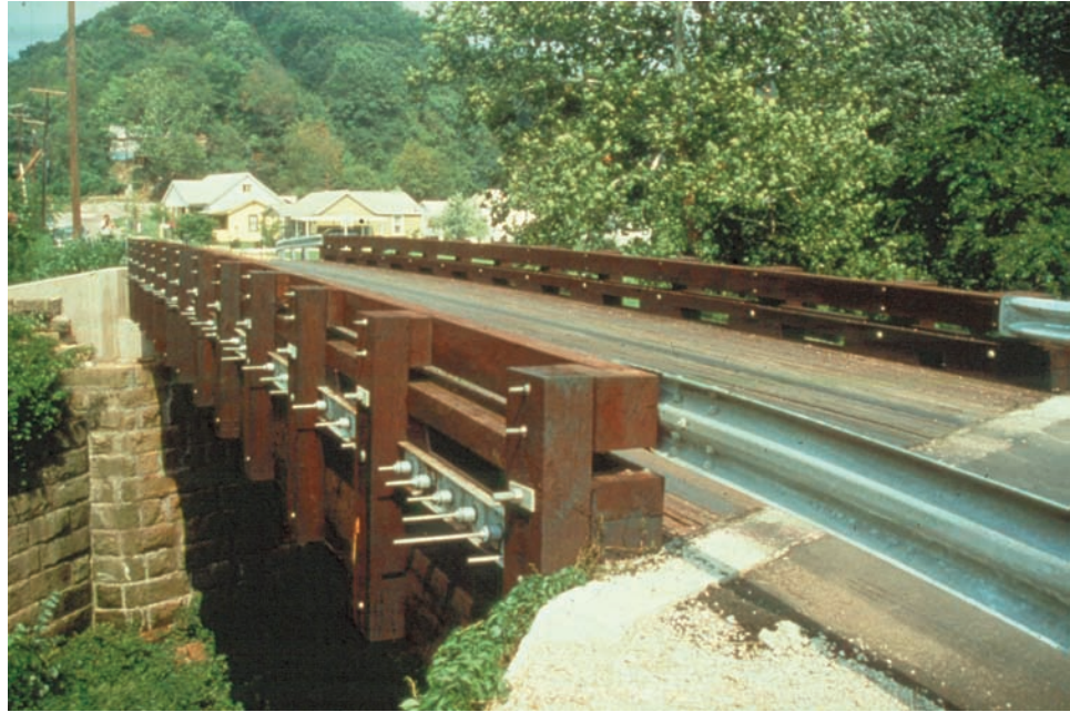
Figure 5.1.4 Stressed-laminated Deck
