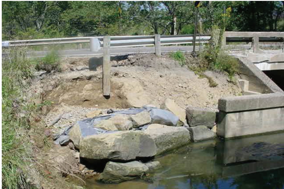
Figure 5.5.12 Erosion Reducing Post Embedment
