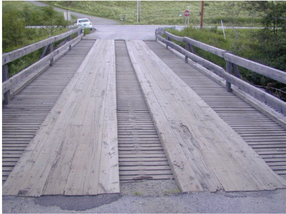
Figure 5.1.6 Timber Wearing Surface on a Timber Deck
