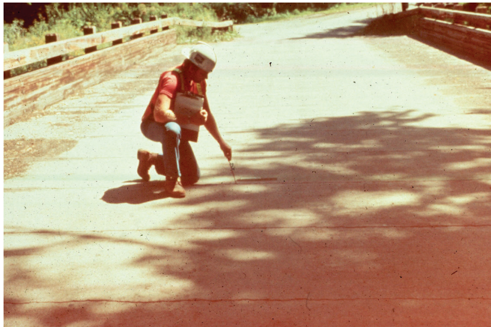
Figure 5.1.7 Inspector Probing Timber with a Pick at Reflective Cracks in the Asphalt Wearing Surface
