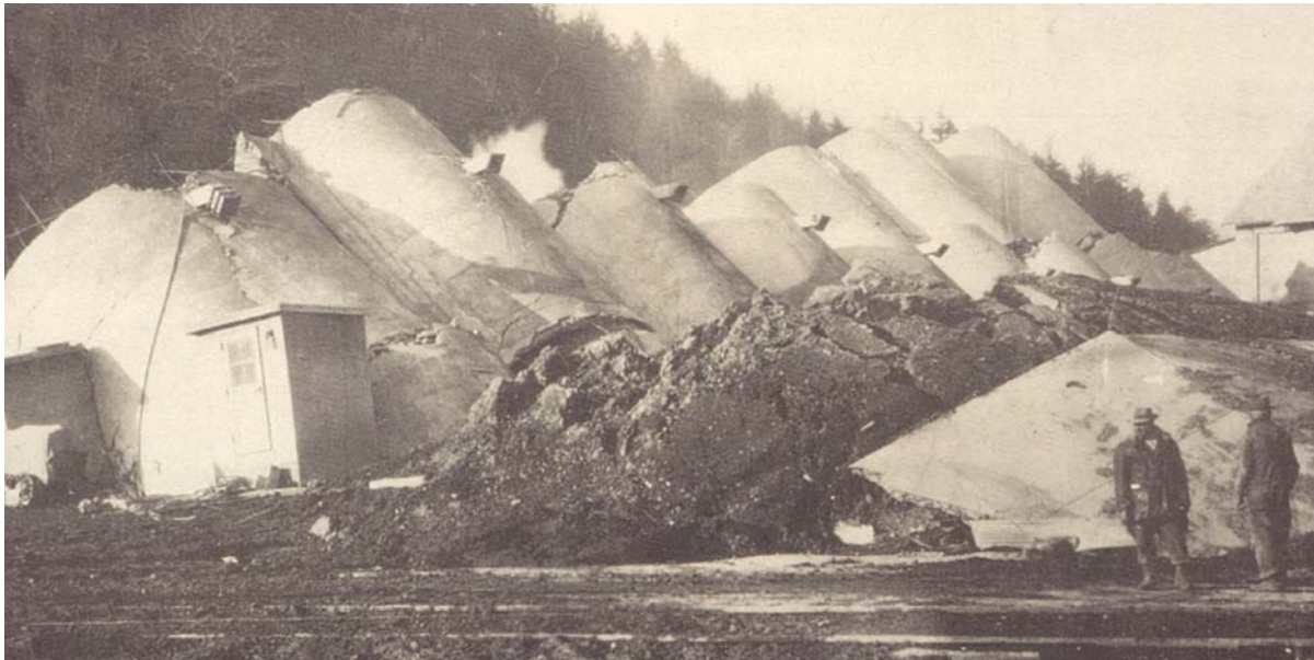
Figure 8-12. Bearing capacity failure of silo foundation (Tschebotarioff, 1951).
