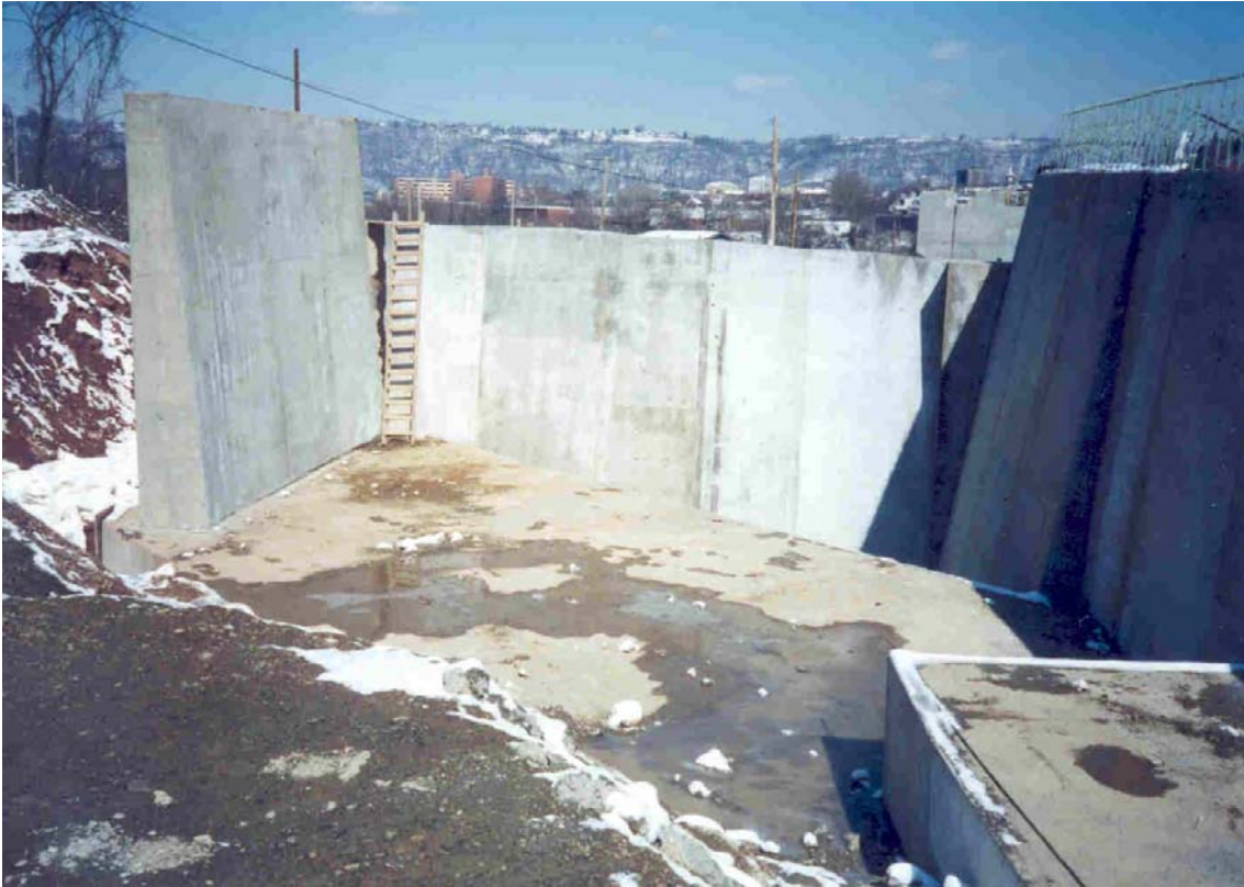
Figure 10-18. CIP abutment with integral wingwalls
