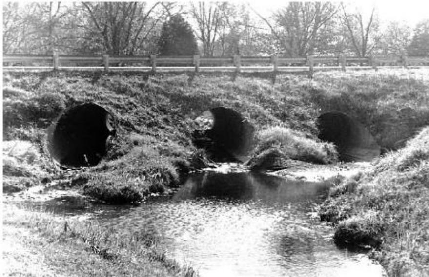
Figure 8 Corrugated Metal Arch Culvert
