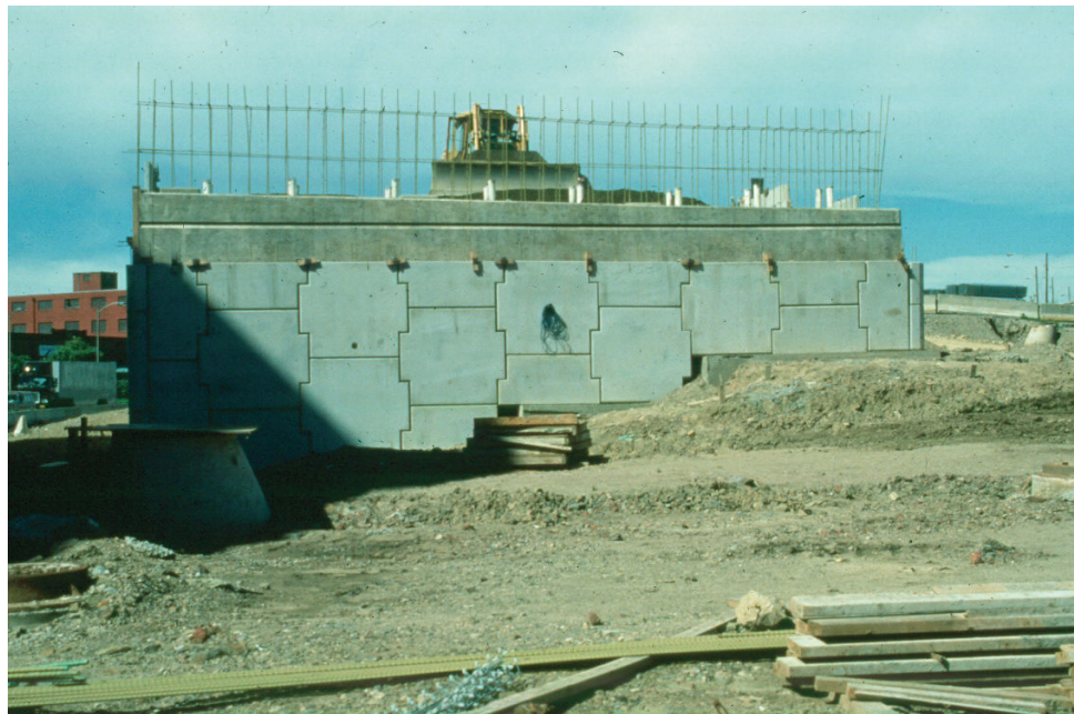
Figure 10.1.8 Mechanically Stabilized Earth Abutment (Note Precast Concrete Panels)
