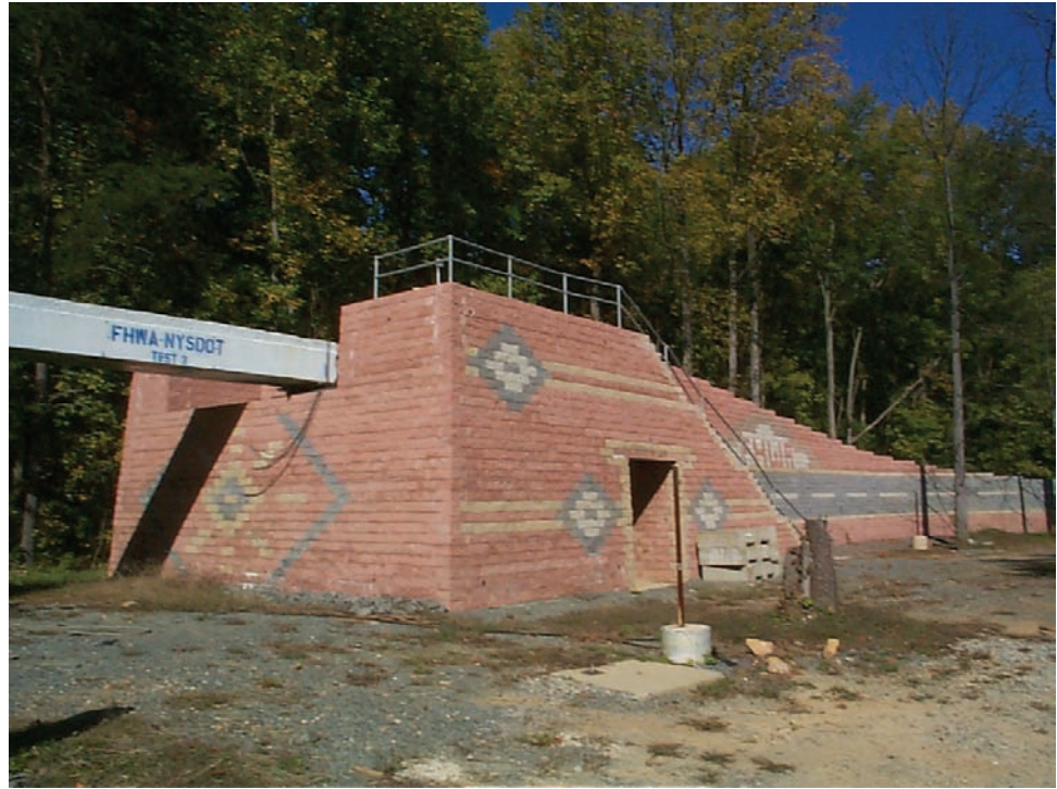
Figure 10.1.10 GRS Bridge Abutment Developed at the Turner-Fairbank Highway Research Center
