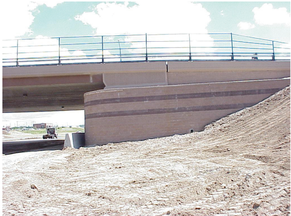
Figure 10.1.11 View of the Founders/Meadows Bridge Supported by GRS Abutments
