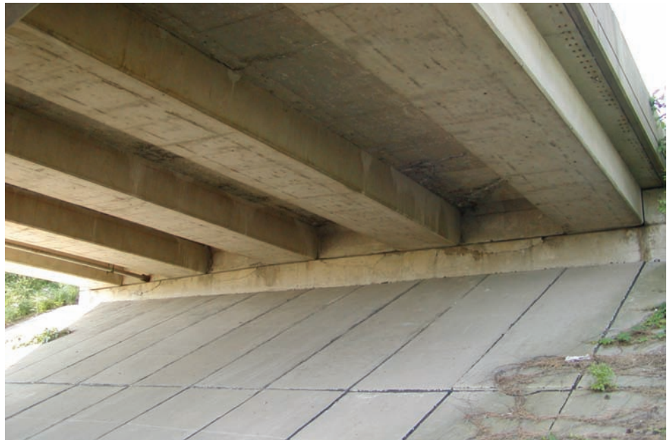
Figure 10.1.4 Stub Abutment
