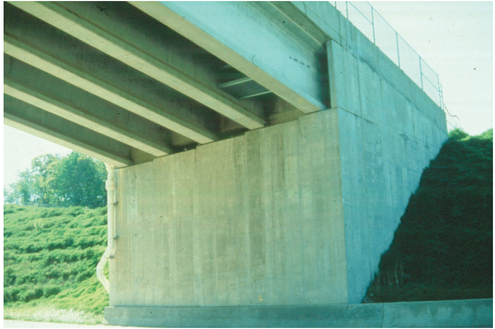
Figure 10.1.3 Full Height Abutment
